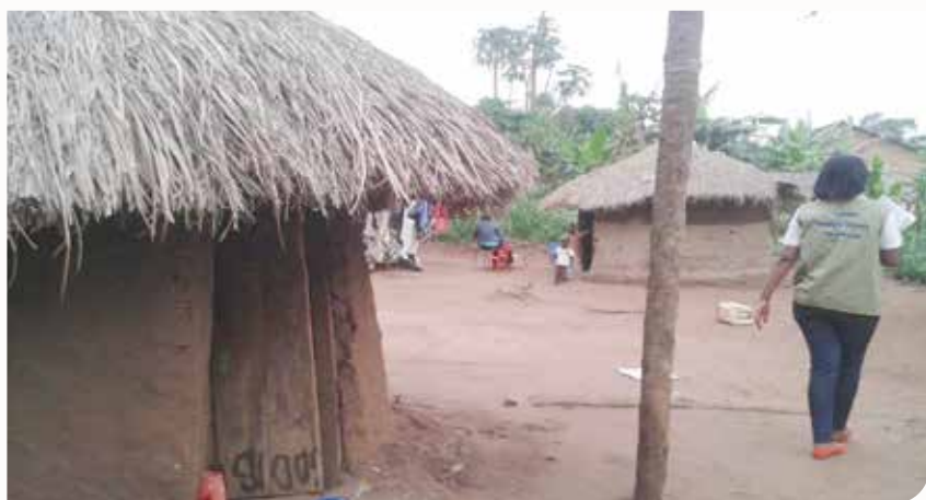
Staff houses at Kikonda Police post in Kyakwanzi District
