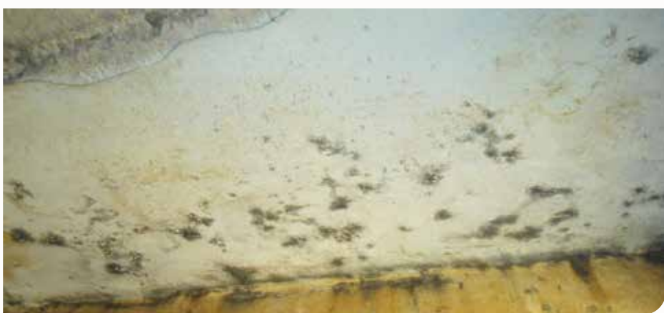
A dilapidated cell with bedbugs at Gulu CPS.
