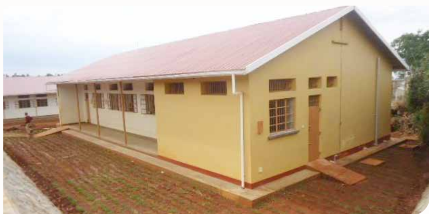
Newly constructed wards at Kapchorwa Prison
