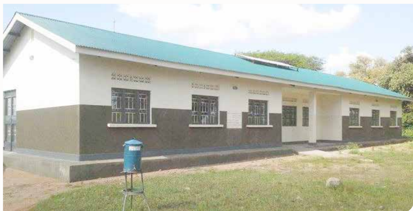
A newly constructed Health Centre III at Lobule Refugee Settlement Camp, Koboko District after being commissioned in 2014 by Hon Hillary Onek, the Minister for Disaster Preparedness and Refugees
