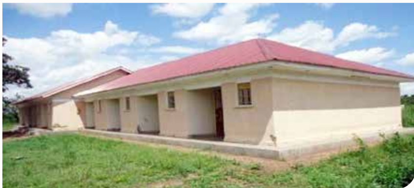
Newly constructed Abuk Police Post in Abim District
