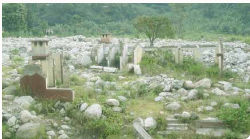
Some the Kilembe hospital staff accommodation destroyed by River Nyamwanba.
