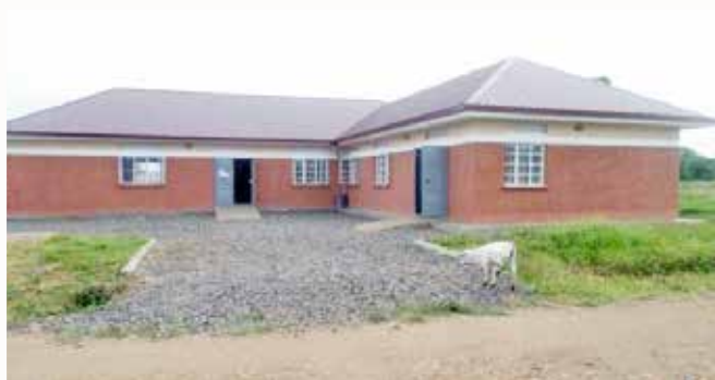
Newly constructed Panyimur HC III in Nebbi District with ramps
